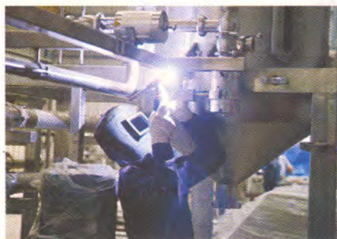
Welding in progress
